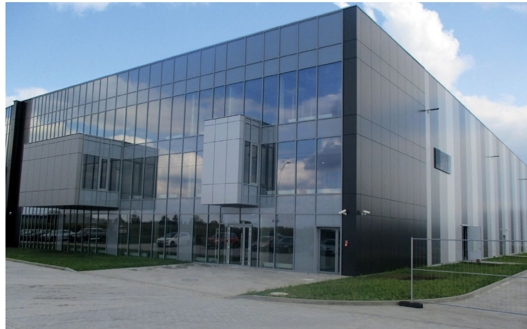
EXTENSION OF THE OLEOPHARM PLANT
