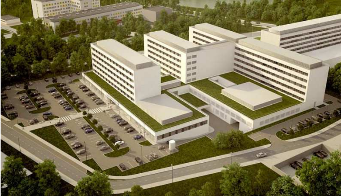
Multidisciplinary Hospital in Katowice
