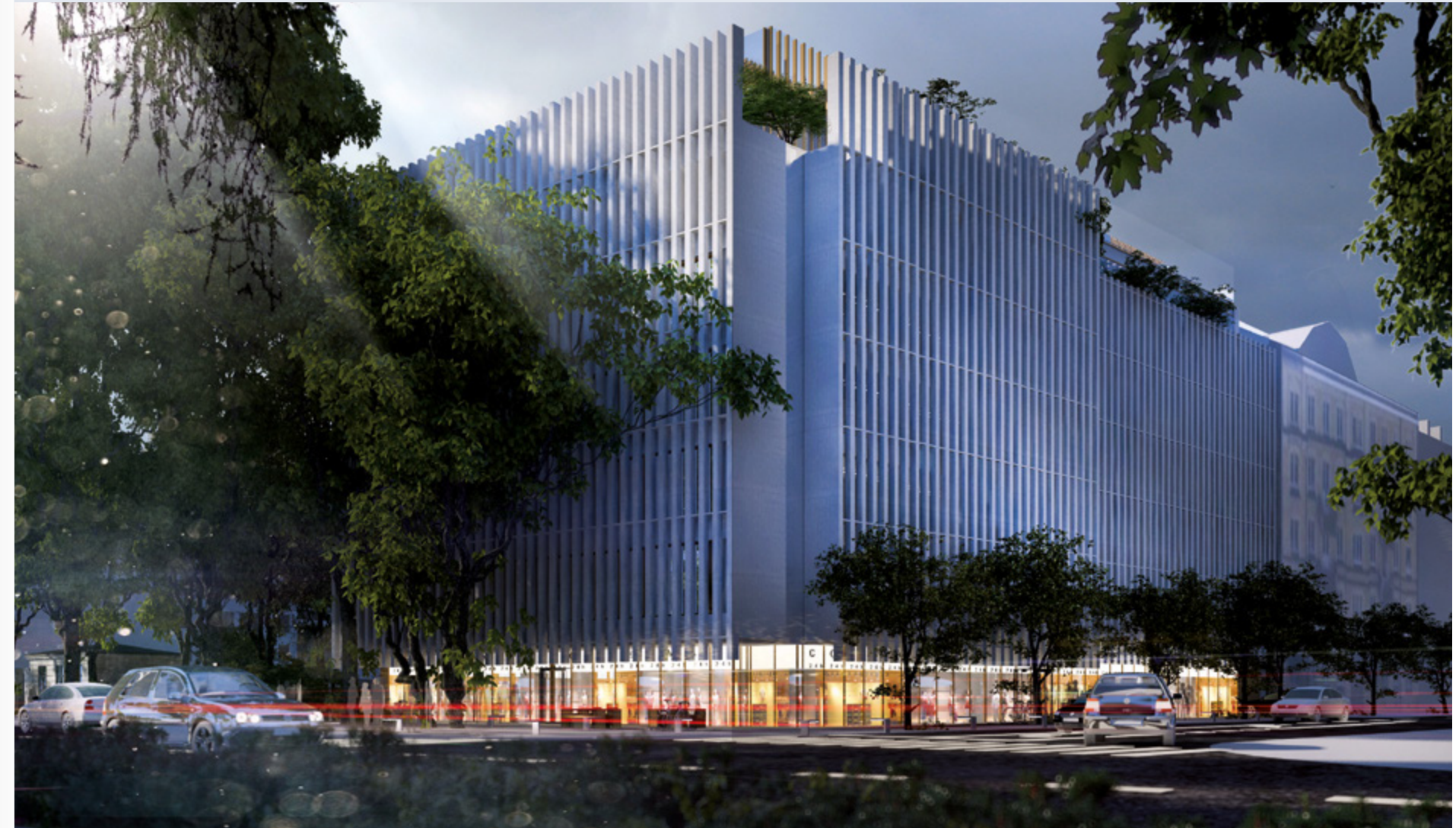
THE "SZUCHA PREMIUM OFFICES" OFFICE BUILDING
