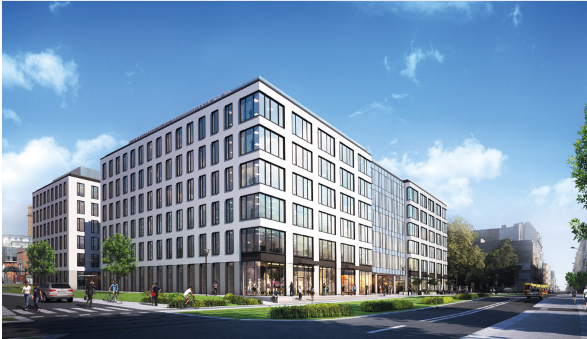
"MBANK STOP" OFFICE AND CONFERENCE CENTER
